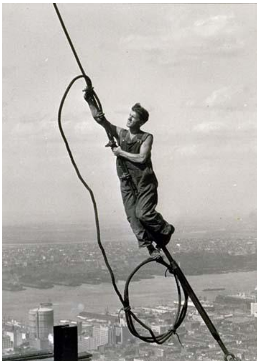
Slika br. 39. Lewis Hine, Gradnja Empire State Building , 1930. https://www.uic.edu/depts/oeo/susi/research_hinesequence.html
