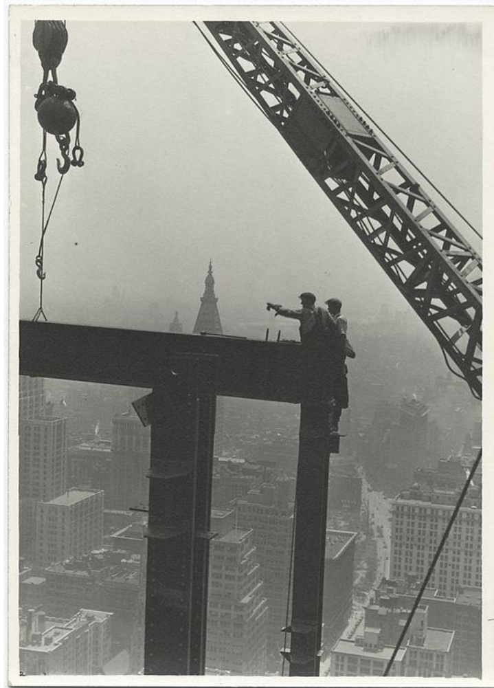
Slika 1. Lewis Wickes Hine, Radnici tijekom gradnje Empire State Building http://www.equipmentworld.com/amazing-empire-state-building-construction-photos-from-1931-show-workers-hanging-on-for-dear-life/#sthash.eMAIpIQY.dpuf
